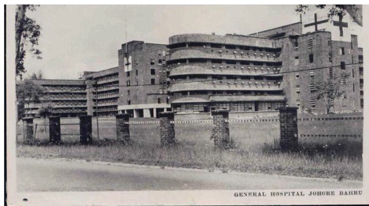
Figure 47. An old photo of Johor Bahru General Hospital
