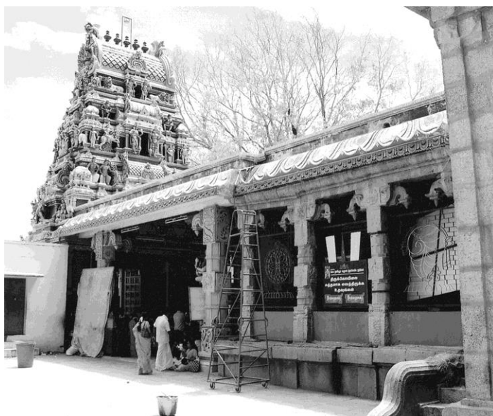
Figure 9. Structural additions to the Āṅaimalai cave temple for Nṛsiṃha.
